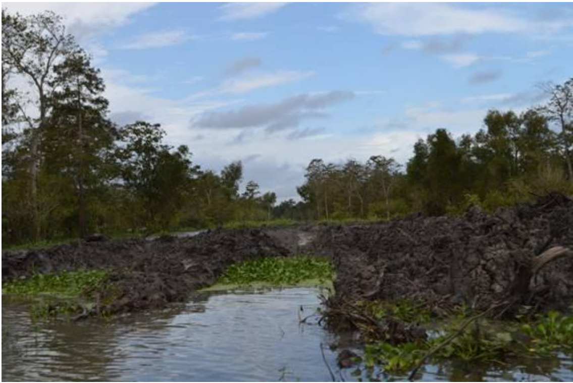
Spoil bank, no gaps
