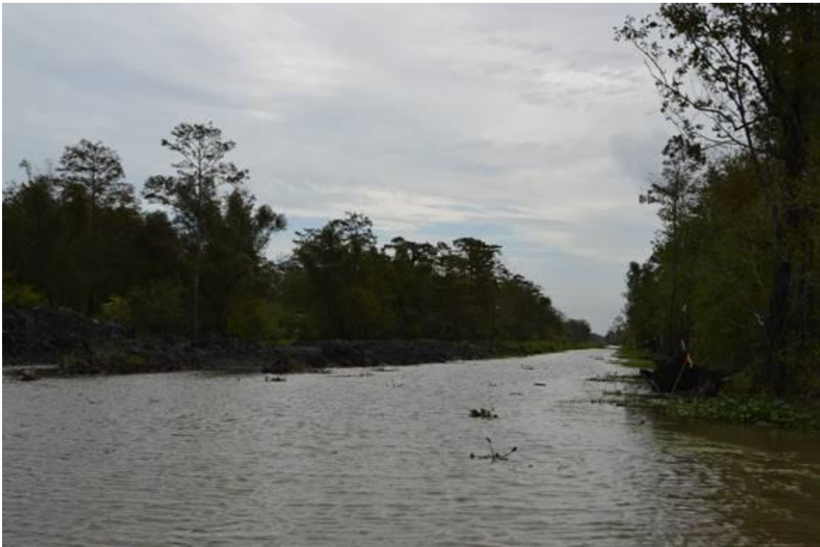
Unnamed bayou dam
